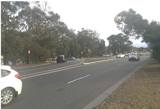
Figure 2.8: New Line Road (looking north)
