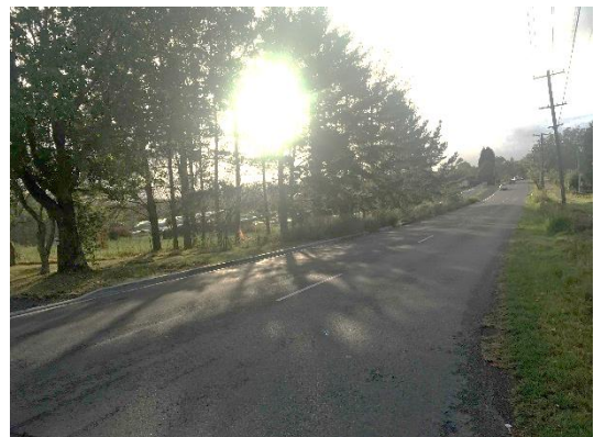
Figure 2.5: Quarry Road (looking southeast)
