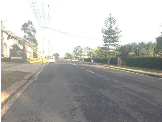
Figure 2.4: Quarry Road (looking northwest)
