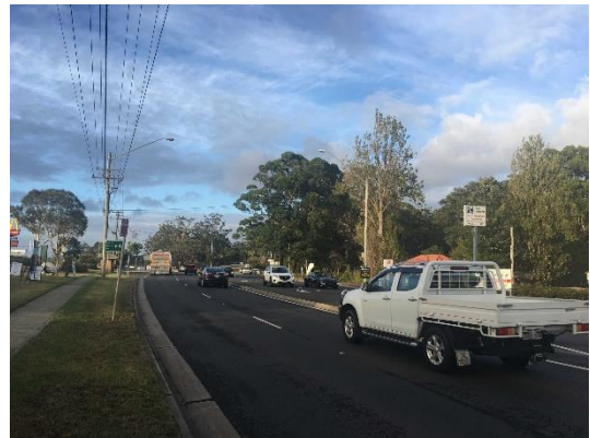
Figure 2.3: Old Northern Road (looking south)
