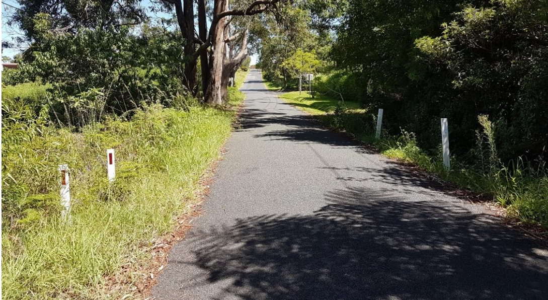
Figure 6.9: Culvert located on Vineys Road
